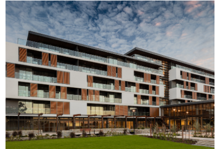
Swan Christian College Renovation 381 Great Northern Hwy, Middle Swan
