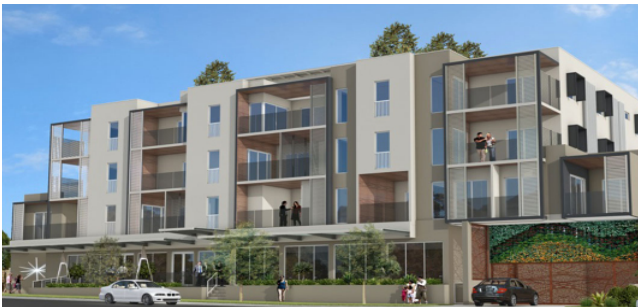
Thomas Building Marmion Street, Booragoon
