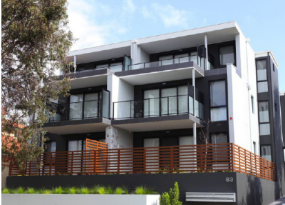
Maylands Apartment 11 Units Over 3 Levels 83 Caledonian Avenue, Maylands
