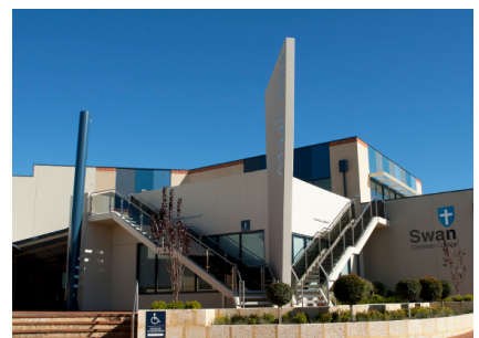
St Ives Retirement Village Renovation 44 Rd Myaree
